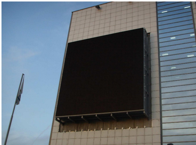
Completed LED display on the wall
