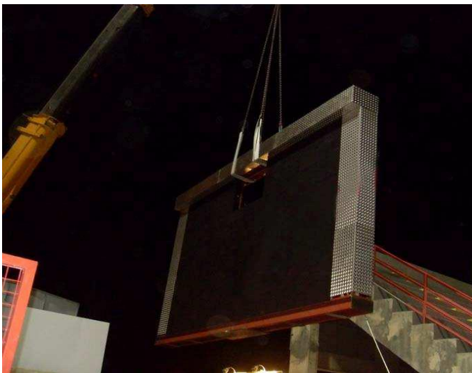
Hanging the LED display up to the roof
